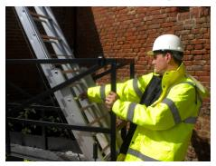
8. Check ladder locks have locked into position.
