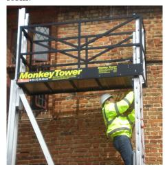
**ADANGER** Do not extend the height of the platform by climbing on the guardrails or using ladders, boxes etc.
